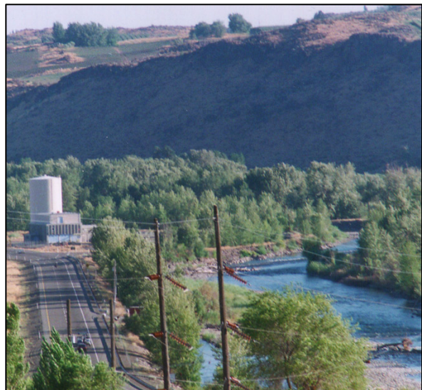
The City of Yakima's Naches River Surface Water Treatment Plant – a possible source of water for recharge in the Ahtanum Valley.
